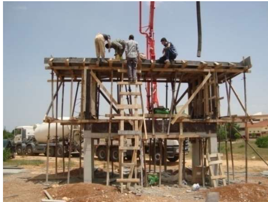
Figure 2: Construction of the experimental full-scale box-girder segment
